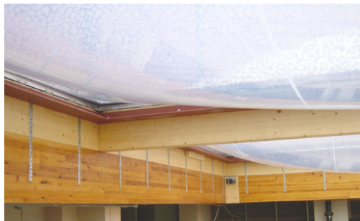
Figure 4.1: Inflated roof lights produced by Buitink technology
