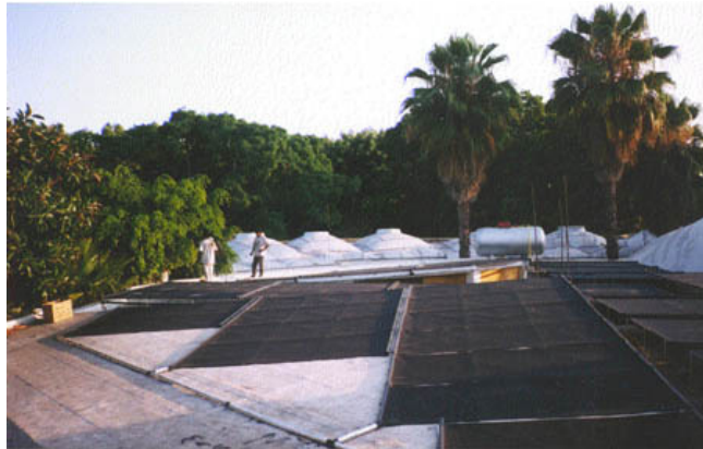
Figure 1.5: Uncovered absorber by Hot Sun industries (ref. 9)
