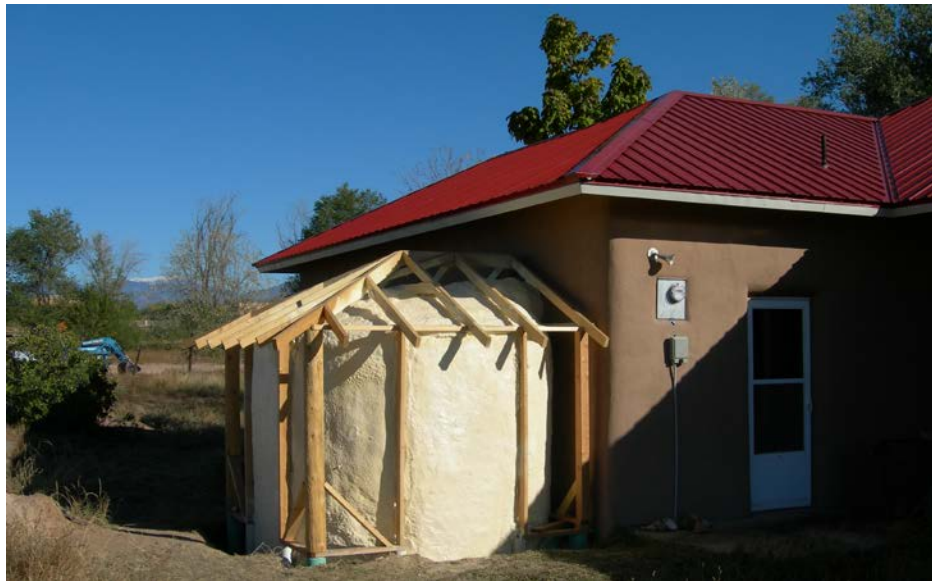
Figure 5. After the foam insulation was sprayed onto the tank.
