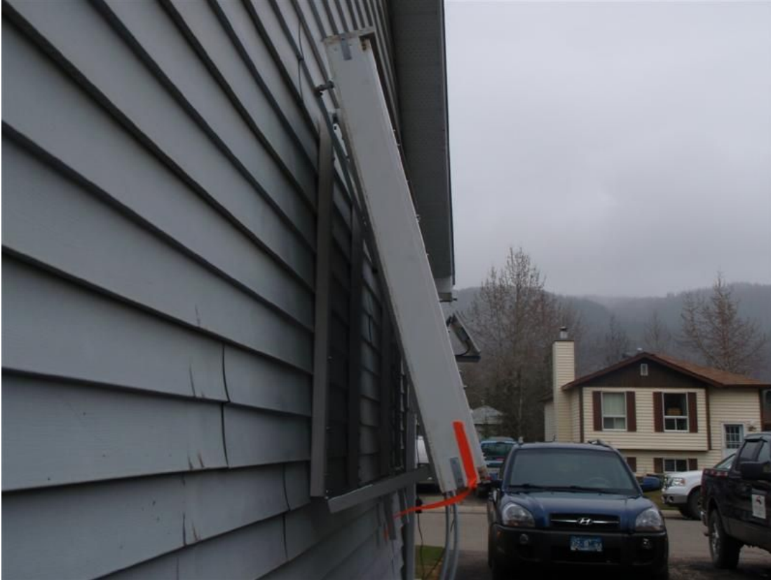
Side view showing the hinged 2 X 4 frame bolted to house
