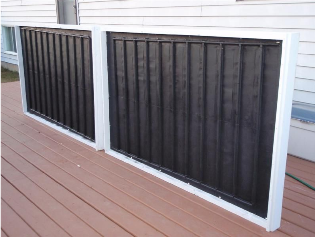
Collectors before glazing went on
