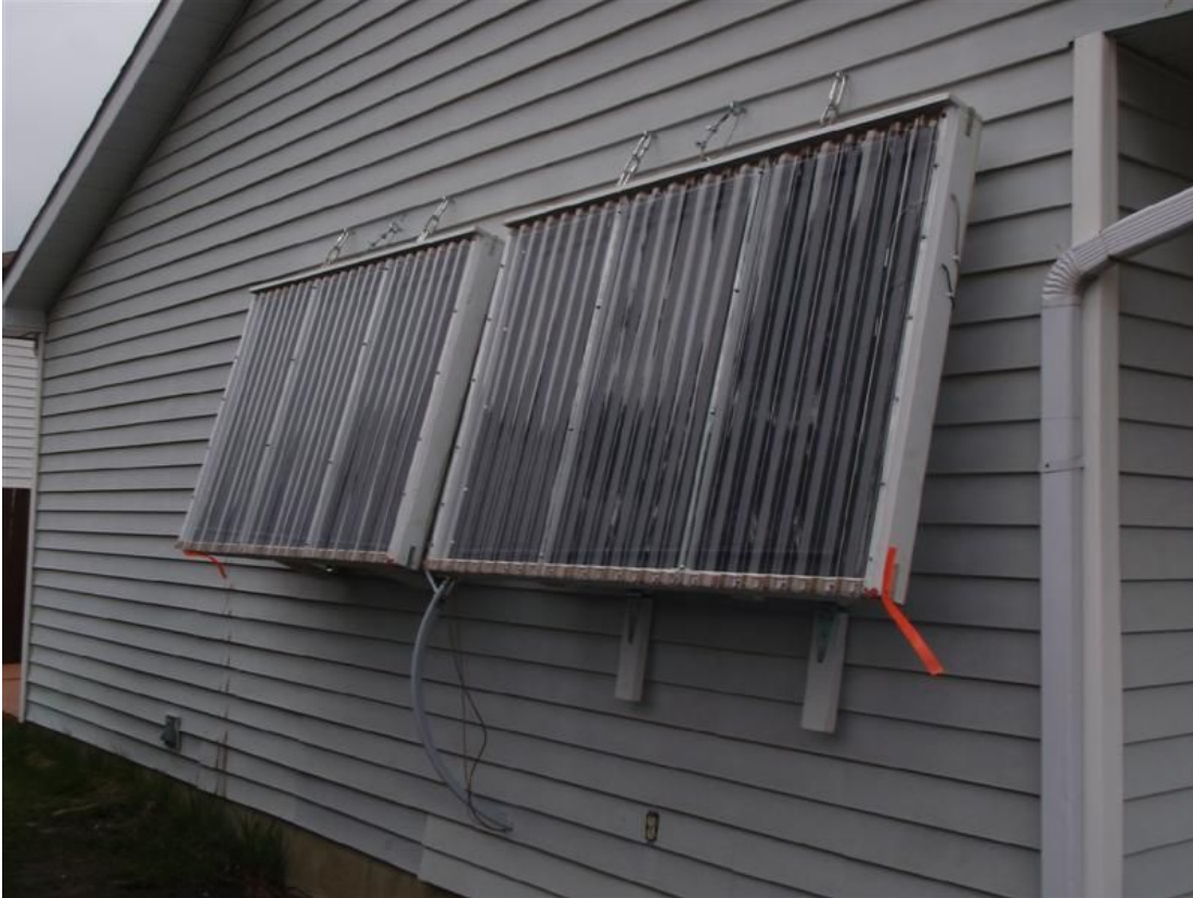
View of the completed collectors
