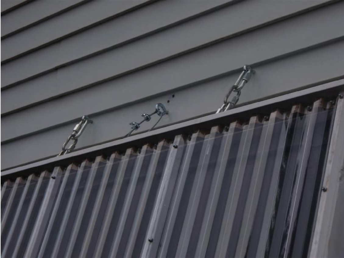
Hangers use screw eyes and quick links
