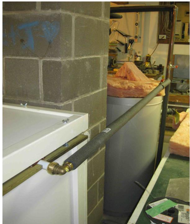
*Illustration 17: Connection between solar tank and existing oil fired water heater.*
