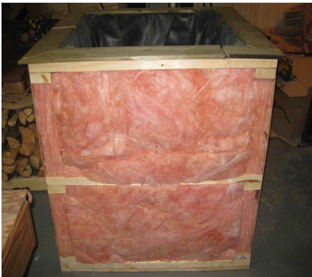
*Illustration 11: R-12 fiberglass batt insulation.*
