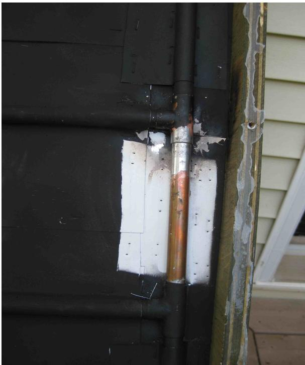
*Illustration 22: The leak site after soldering. It held!*
