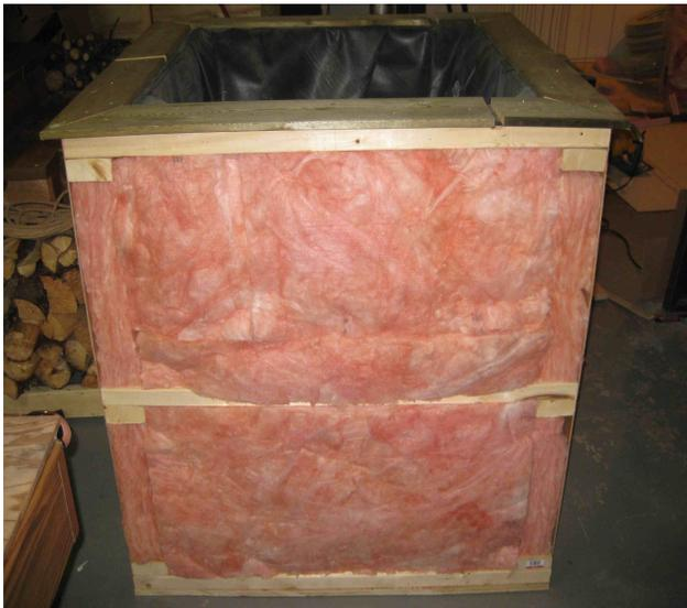
*Illustration 11: R-12 fiberglass batt insulation.*
