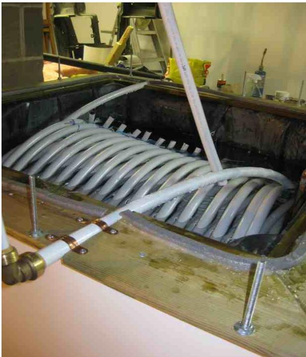
*Illustration 16: Heat exchanger in tank. Inlet pipe is foreground.*
