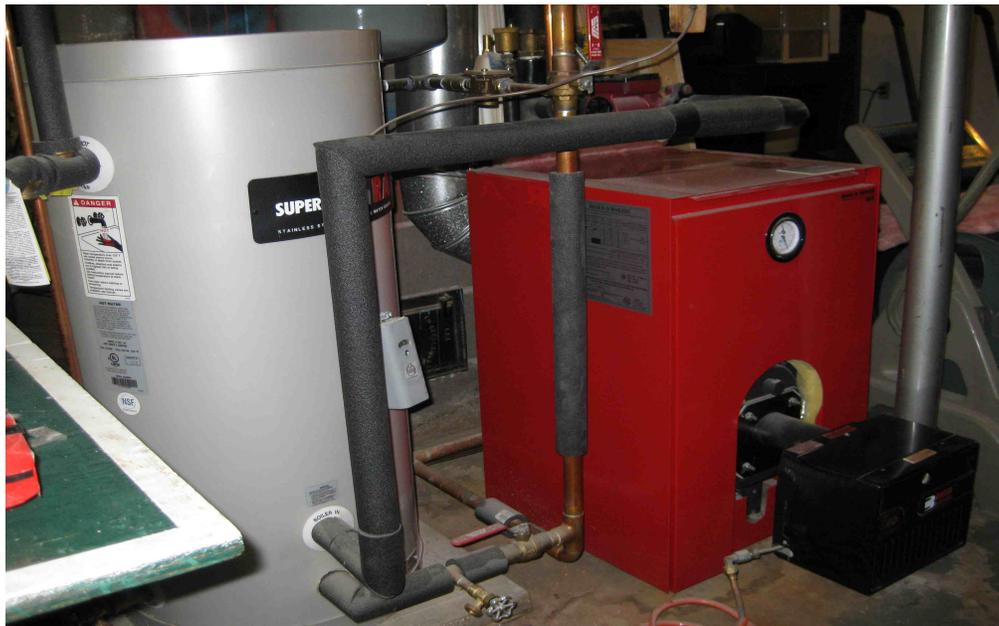
*Illustration 1: The new Biasi high efficiency furnace with a Superstor Ultra indirect 30 gallon water heater cut our heating oil consumption by about 25%*
