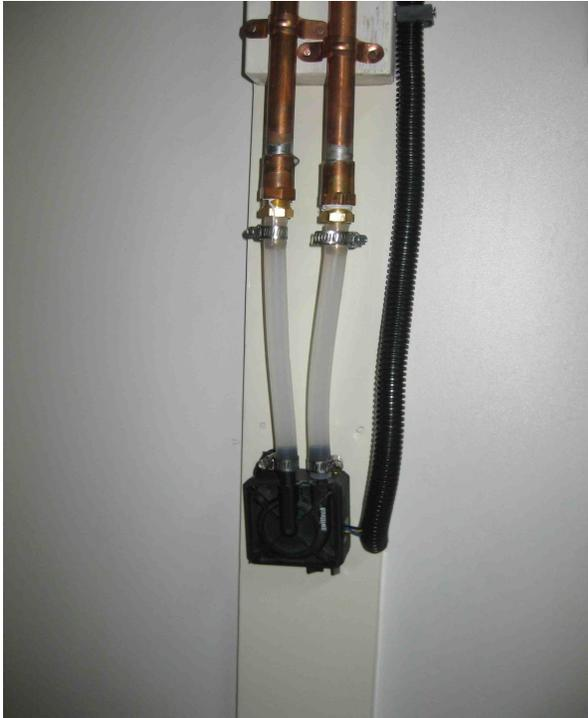
*Illustration 18: Swiftech MCP355 pump uses only 18 watts and is quiet.*
