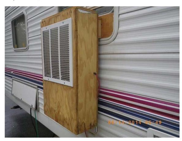
The top of the water can is at the same height as the bottom of the grill. The cooling pad is aspen pad which is commonly used in swamp coolers. I ordered a roll online and cut a piece large enough to cover the opening at the air intake.
