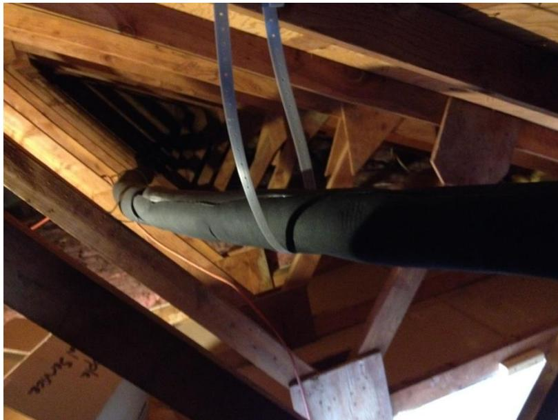
**Return Line Through Crawl Space:** Plastic pipe hangers were used to secure piping. Note that all piping was sloped at all times, especially since this is an unconditioned space.
