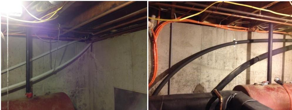
**Supply and Return Lines in Basement:** The picture on the left is before the lines were insulated and supported to the wall. The picture on the right the lines are both insulated and supported. One line feeds into the tank (not shown).
