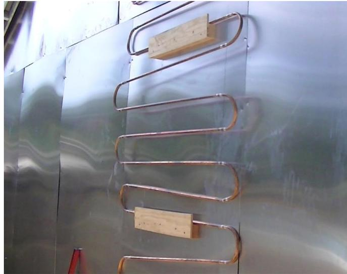
**Mounting the 1<sup>st</sup> Pararrel Circuit:** Wooden hangers in use
