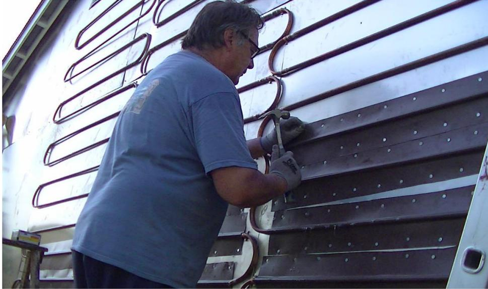
**Securing Fins to Wall:** Roofing nails were used to secure fins to wall. Pre-drilling was necessary to penetrate the aluminum backing.
