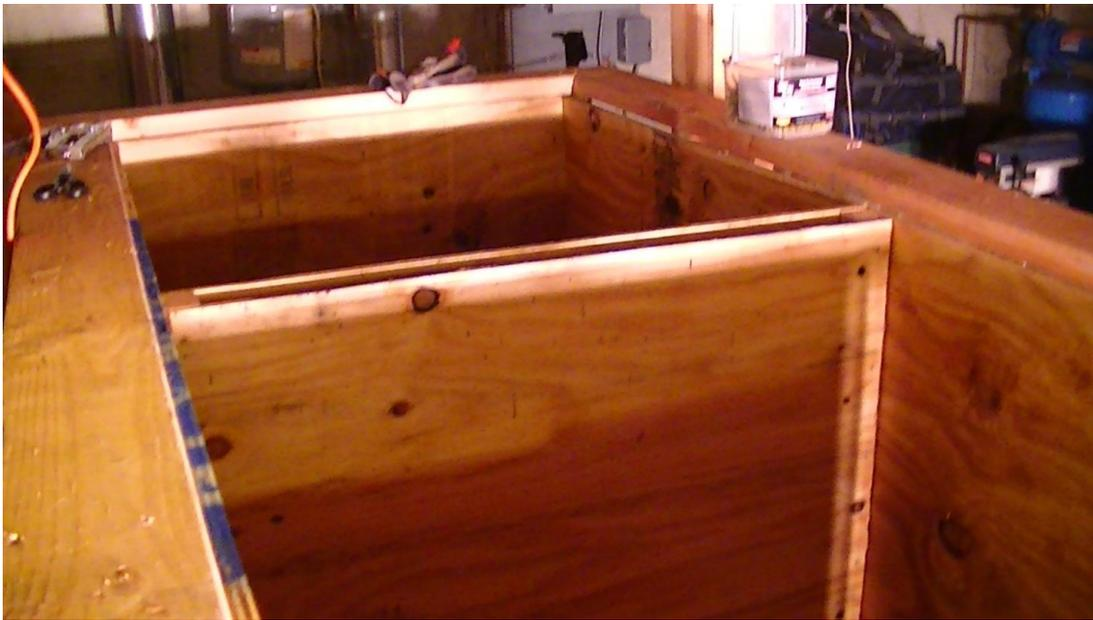
**Top Header and Center Partition in Place:** Tank complete without EPDM liner, sensors and plumbing.
