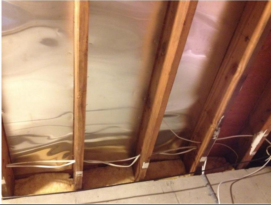
**Flashing Installed Between Floor Joists:**
