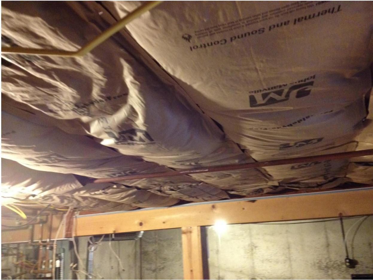
**Insulating Between Floor Joists:** Heat loss from the first floor of the home is minimized by adding batt insulation. This also insures the heat from the radiant floor heating system goes up into the first floor of the home instead of down into the basement.
