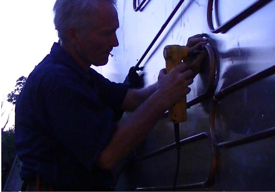
**Securing Circuits with ½ Copper Clamps:**
