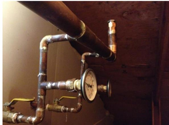
**Top Manifold:** Vacuum breaker shown, note vacuum breaker must be at the high point of the circuit.
