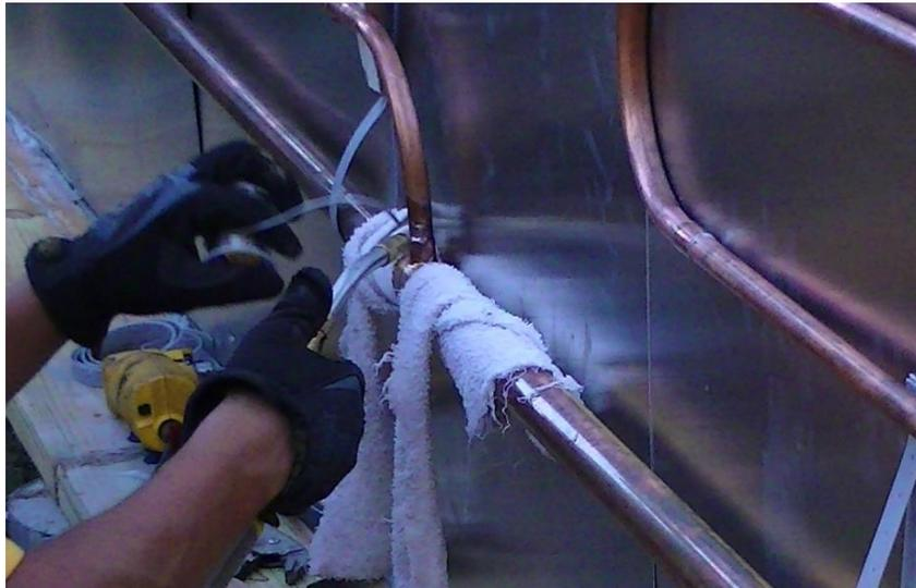
**Soldering a Circuit to the Bottom Manifold:** Wet rags were used so the other solder joints would not come apart.
