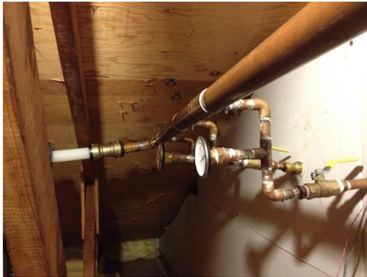
**Top Manifold:** Notice the sloping of the line, the temperature gages, shark bite connection and electric wires for both the temperature sensor and data logger.
