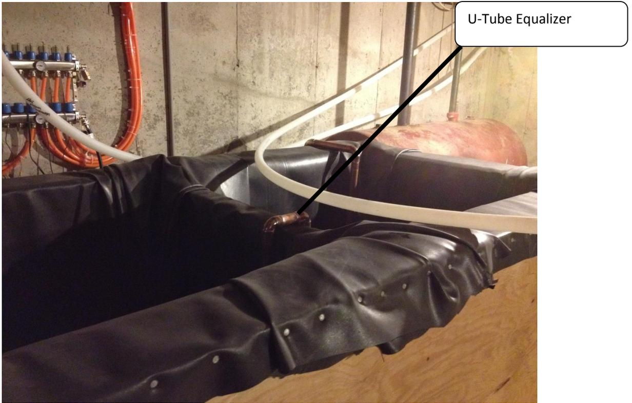
**EPDM Liner and U-TUBE equalizer installed:** EPDM liner tacked onto tank with roofing nails.
