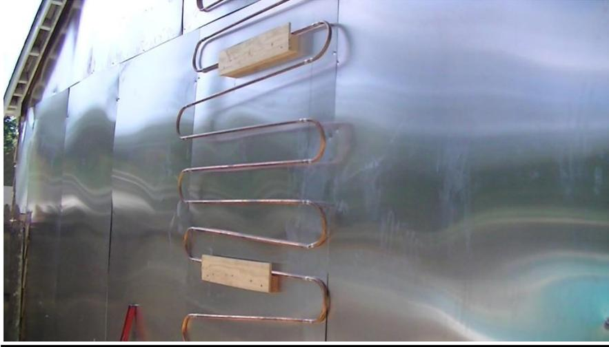
**Aluminum Backing Added to South Wall:** Wooden hangers were made to hang each circuit; this made securing the circuit to the wall much easier.
