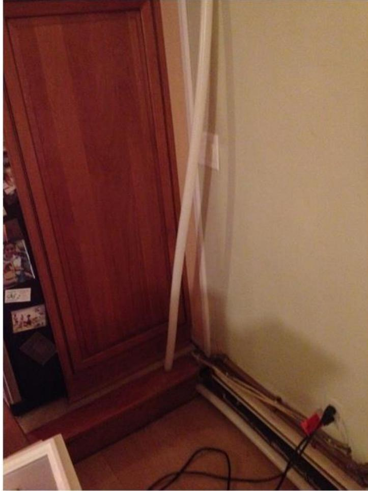
**Supply and Return Lines:** A chase will be built to cover the plumbing. Supply and return lines will also be insulated. The vertical line is the hot return coming from the crawl space. The lower line is the cold supply line feeding the bottom of the collector.
