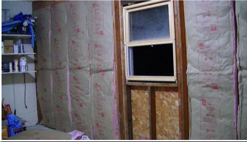
**Fiberglass Insulation Mounted to Most of Wall:**
