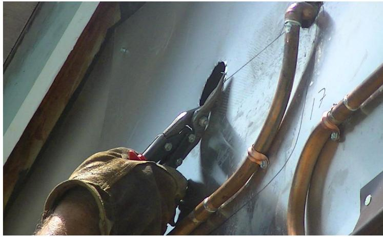
**Tin Snips Used to Enlarge and Clean Up Hole:**
