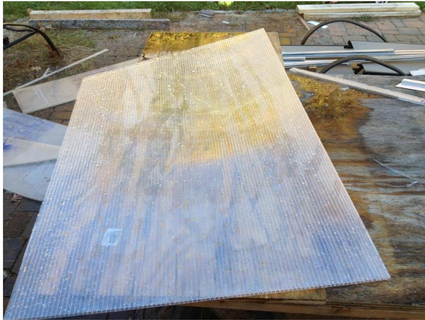
**Polycarbonate Cut on an Angle:** Saw dust and debris would get inside the twin walls, so we used a hose to clean out the polycarbonate before mounting. Moisture would dry out over time.
