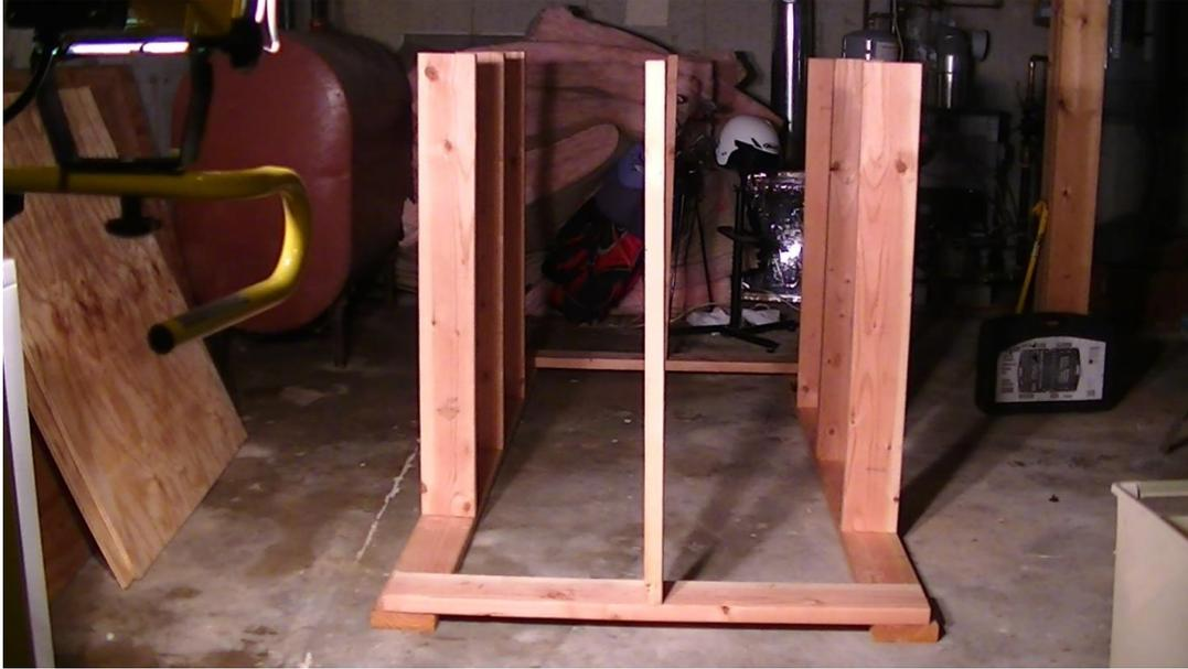
**Bottom Heater and Studs in Place:** Tank built in a similar way to framing a wall.
