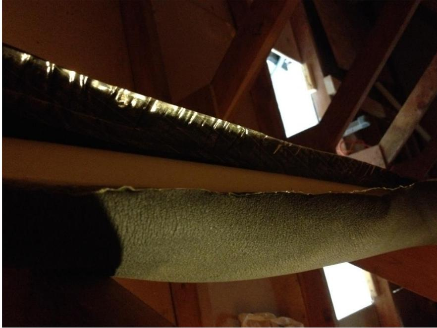
**Insulating the Pipe:** All piping to and from the collector should be insulated, especially the hot (return) line. Insulating was easy; just remove the adhesive tape and touch the tabs together.
