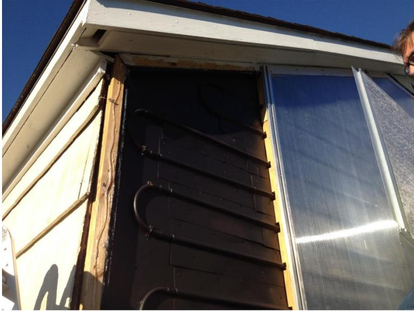
**Adding the Last Piece of Twin Wall Polycarbonate:** Note the heavy bead of silicon along the perimeter.
