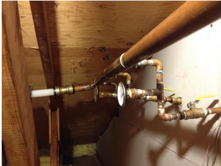
**Copper to PEX Transition:** All copper to PEX transitions were performed using shark bite Connectors.
