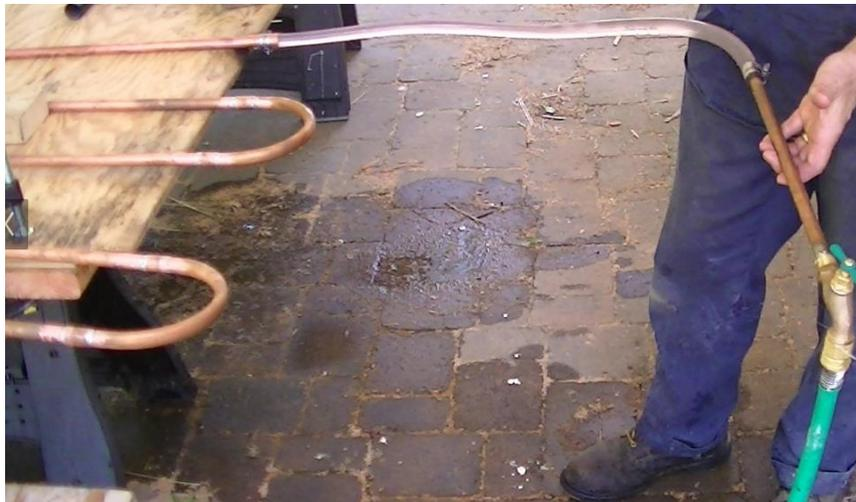
**Hooking the Hose to the Copper Circuit:** A straight piece of copper piping was soldered to a hose bib. Inexpensive C-Clamps were obtained from the hardware store, with some plastic tubing to allow for easy on / off method for leak testing.
