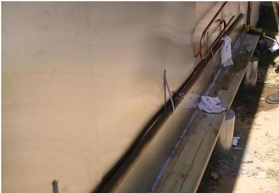
**Mounting Bottom manifold:** Plastic pipe hangers were used to temporarily secure the bottom manifold. They were eventually replaced with metal pipe hangers because the collector would be too hot for the plastic. Plastic hangers were a good low cost and temporary support system.
