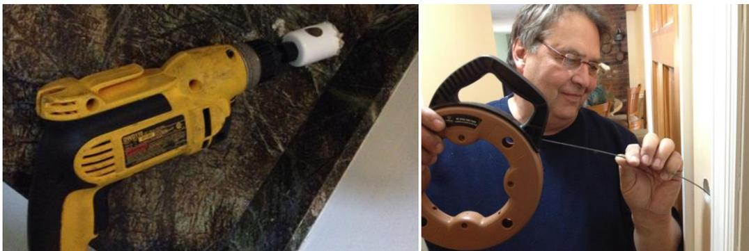
Snaking the Wire through the Wall Into the Basement: Use 1 inch hole saw to drill through the dry wall. Tape the electrical wire to the snake and feed through the wall into the basement.
