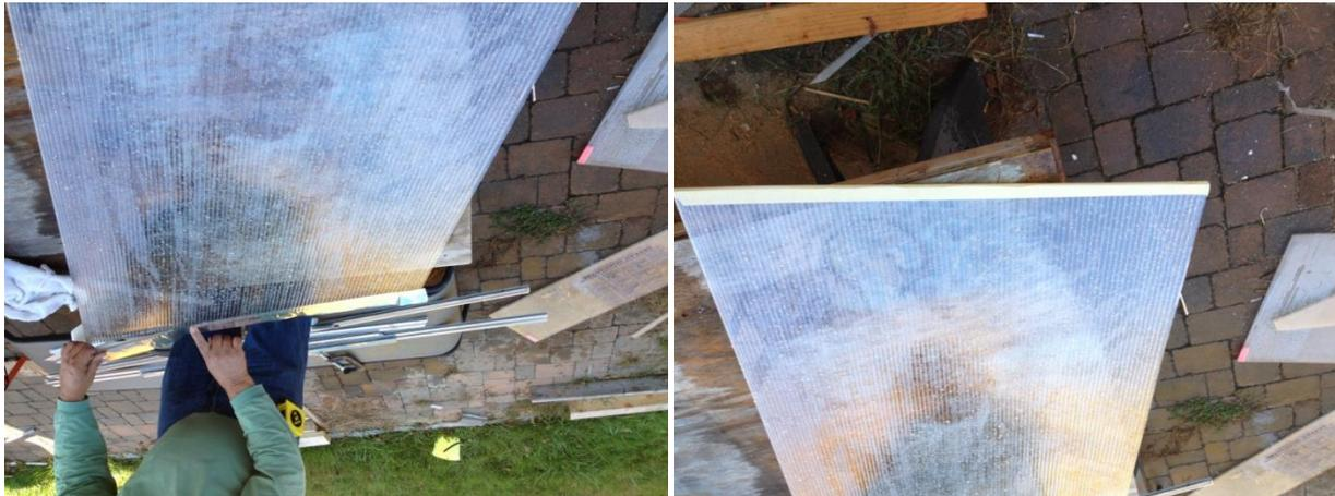
**Aluminum and cloth tape added to top and bottom of polycarbonate respectively:**
