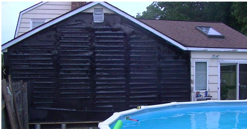
**South Wall Complete and Painted:** The only step remaining on the wall is the twin wall polycarbonate
