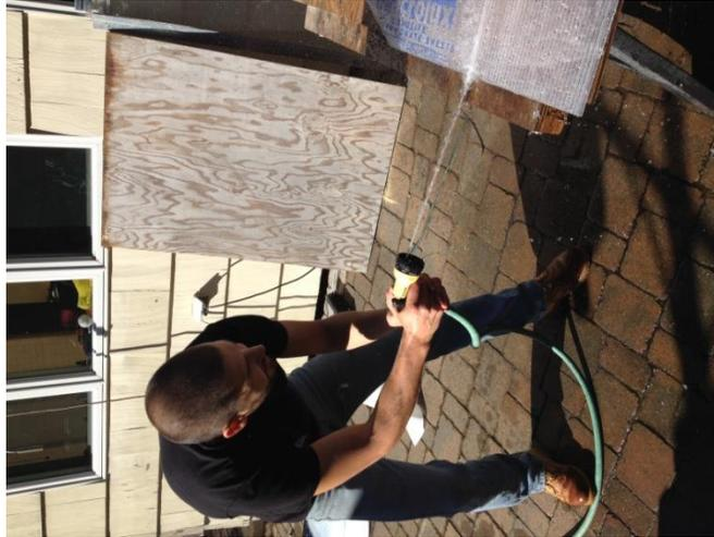
**Hose with a Nozzle used to Clean Polycarbonate after Cutting:**
