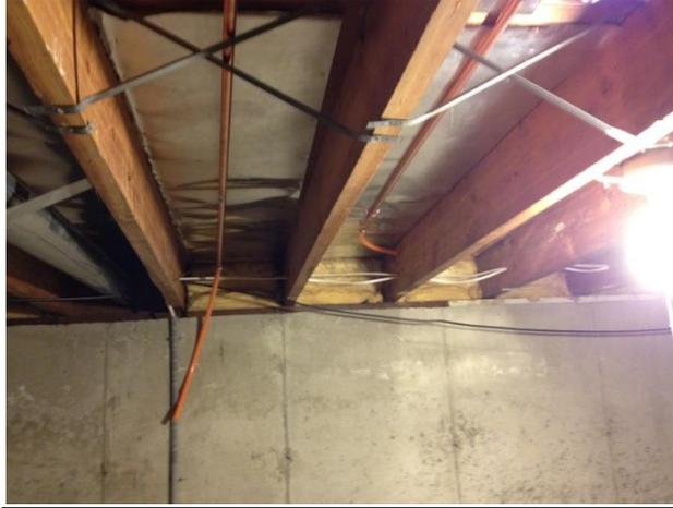
**Installing the Copper Between the Floor Joists:** Note the PEX transitions around the bends.
