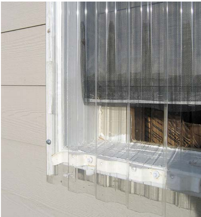
A close view of the lower sill, lower vent, left end's vertical glazing supports, and screen absorber. "Wiggle" closure strips secured to the sill plates help seal the glazing panels.
