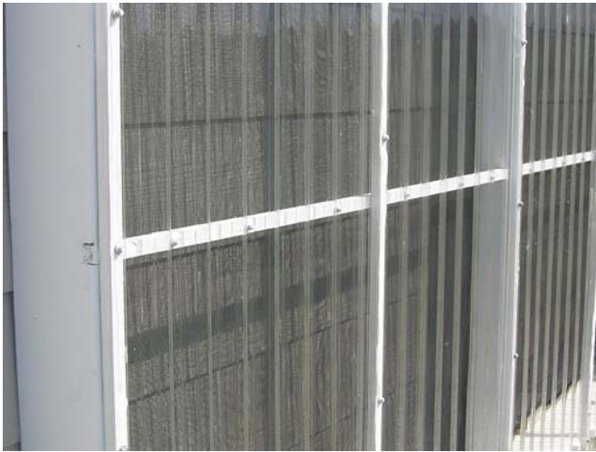
Horizontal support strips run along the back side of the corrugated panel sections. Vertical strips inside the corrugations tie the panel sections together.
