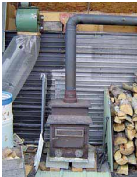
A wood stove supplements heat in cold weather. Heat from the stove is circulated to the greenhouse by a furnace fan that blows the hot air through a poly duct.
