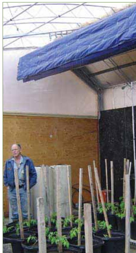
Interior thermal blanket at one end of the other solar greenhouse at St. Francis Xavier.
