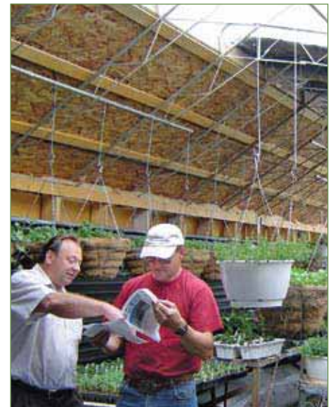
The steel ribs, the sand-filled rear wall, and sloping section of wall shown here are all standard features of the solar greenhouse at Ashern. Steel ribs are handy for hanging plants. The sloping section of wall will be clad in white or silver roofing tin to reflect sunlight onto the plants.
