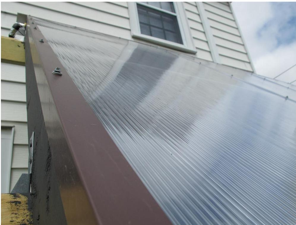
The sides and top of the polycarb sheets are screwed directly into the frames (using screws with rubber washers also sold with the polycarb sheets). Then I bent some aluminum flashing to cover the entire top of the collector and sides halfway down. This gives the collector a more finished look and will protect the wooden collector frame (I also painted this with black deck stain).
