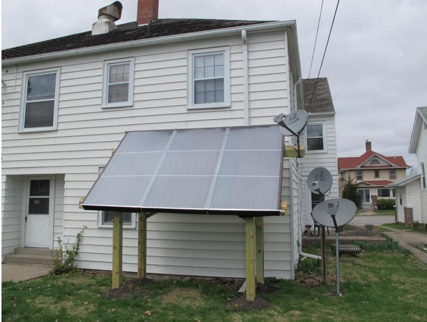
This ground-mounted drainback system follows the design and build instructions from Gary’s site with a few minor exceptions. The system provides an undetermined percentage of the domestic hot water for a seven-unit apartment building in Southeastern Iowa (41 degrees latitude).
