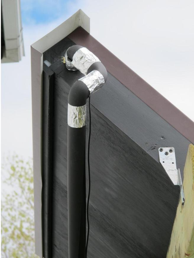
I soldered the  $\frac{3}{4}$ " manifolds parallel to the frame of the collector. To get the needed slope for drainback, the ground mounted rack is sloped  $\frac{1}{4}$ " per foot.
