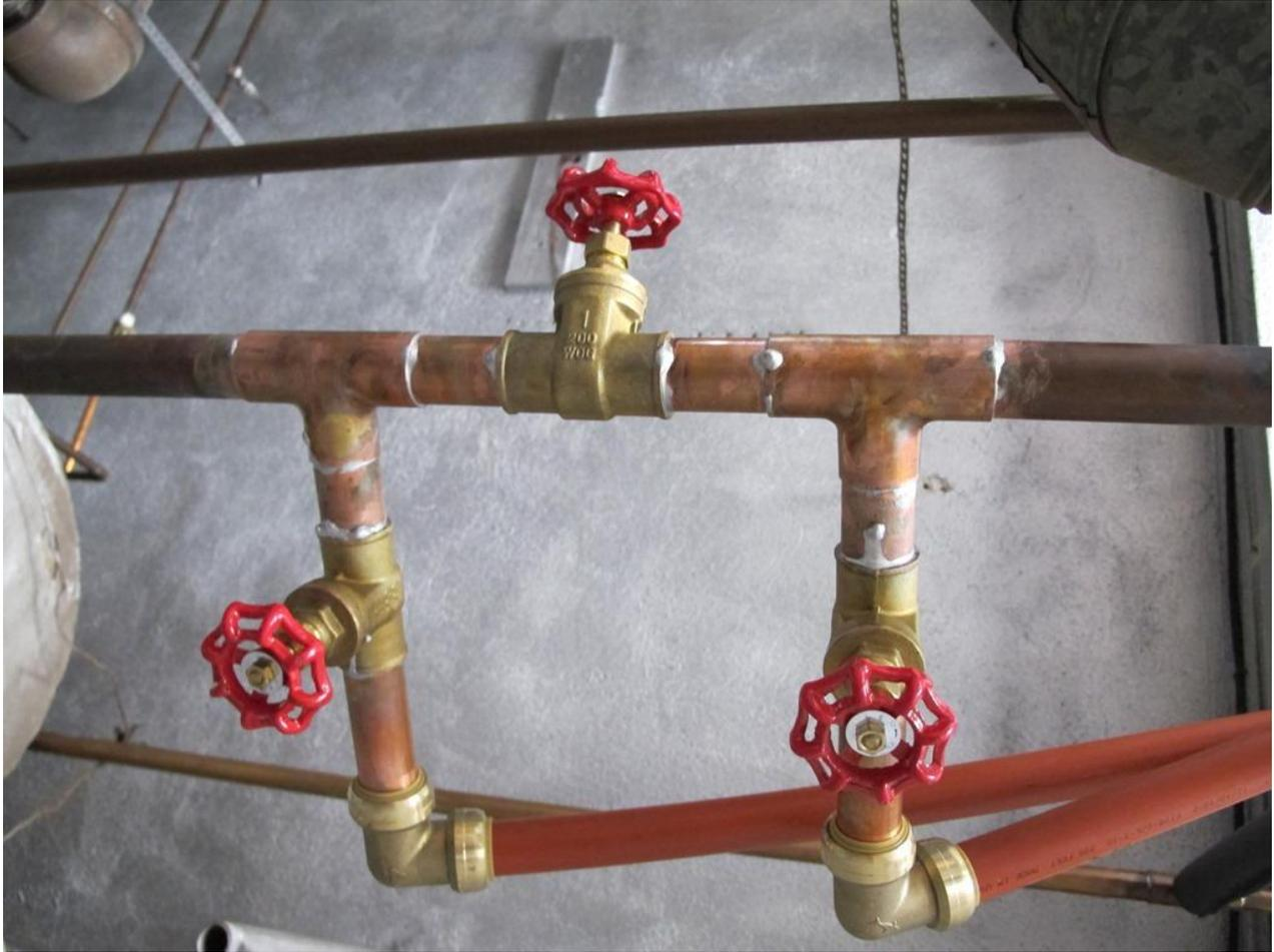
The buildings 1" copper cold water inlet. Bottom valves, Sharkbite elbows and PEX connect to the heat exchanger in the tank.
