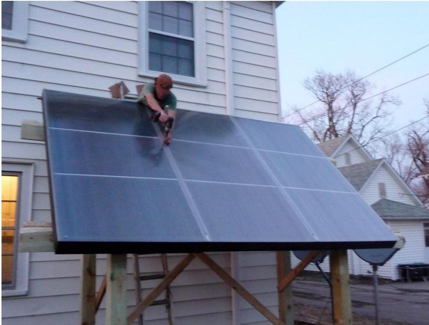
I joined the 6mm twin-wall polycarbonate sheets using purpose made joiner strips sold right alongside the sheets in Menards. They work nicely because they have a ¼” space perfect for screwing the joiner to the collector frame. The hardest part in using them was getting the sheets into the slot. We ended up needing to use a silicone spray lubricant.
