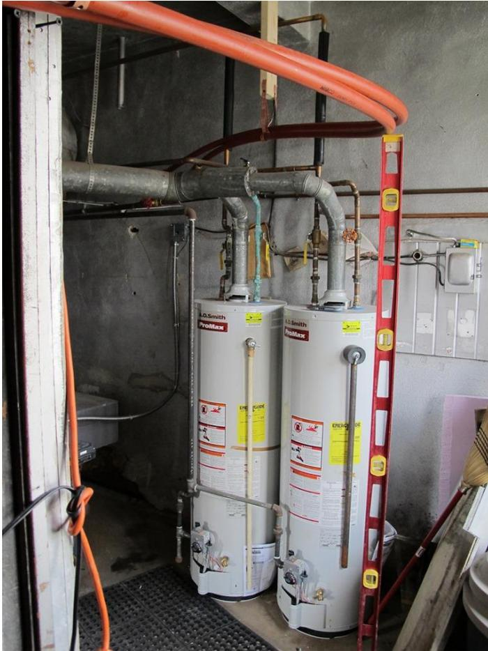
The two natural gas water heaters now supplemented with solar heat. An interesting thing I discovered during the construction was that the solar tank alone provides a boost of 10F to the incoming cold water. Water comes from the mains at 55F and leaves the solar tank heat exchanger at 65F with no collectors attached. The utility room stays very warm because of heat given off by a large boiler system that heats the building and the gas water heater flues.
