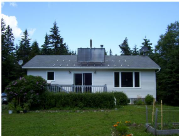
After doing a simplified spreadsheet analysis of heat losses in the collector I decided to go with twin wall polycarbonate glazing of 10 mm or 3/8 inch on the front and 2 inches of polyiso insulation behind. Both these were difficult to obtain where I live (New Brunswick, Canada). In fact to get a reasonable price on the glazing, I bought it in Ottawa (1200Km away) while on a family trip and brought 5 sheets of it back on my cars roof rack.
