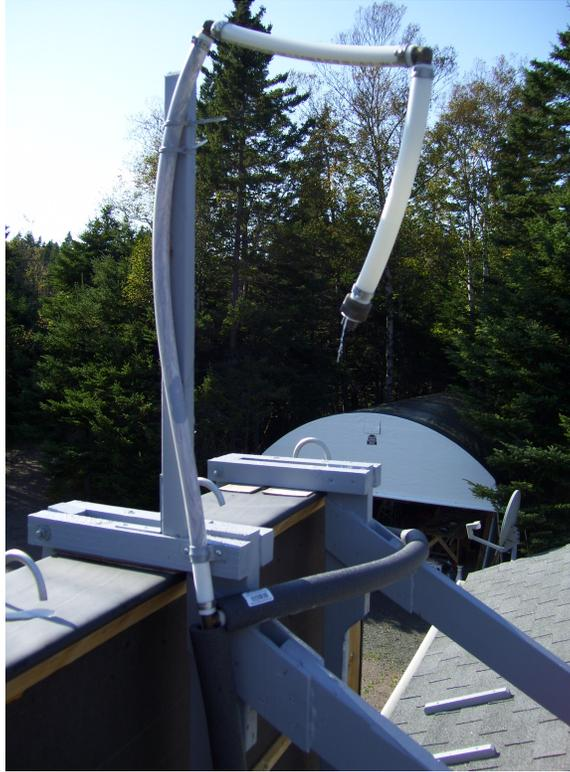
The air trap is just a tee mounted at the highest point of the plumbing with a straight vertical pipe and two 90 degree elbows. Any air in the system bubbles up into the straight pipe and stops circulating back to the pump.
