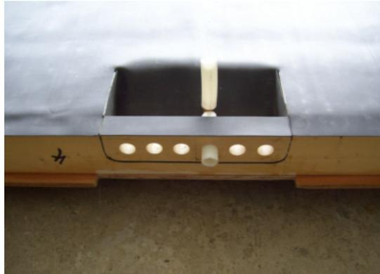
Underneath the tank is a pan made of EPDM rubber and has a drain tube in its corner. Should the tank ever leak I hope the pan will catch the water and we will be able to pump it out to a basement drain.
