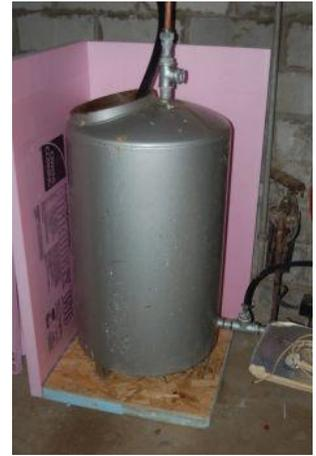
Because this tank is steel and I did not have to use the EPDM that Gary used I didn't feel I needed to limit my temperature. I am also concerned about the effects of high temperature and moisture on the wood in the panels. Therefore one of the changes I made to the original design was to use the track for steel studs for the frame of the panels instead of wood.
